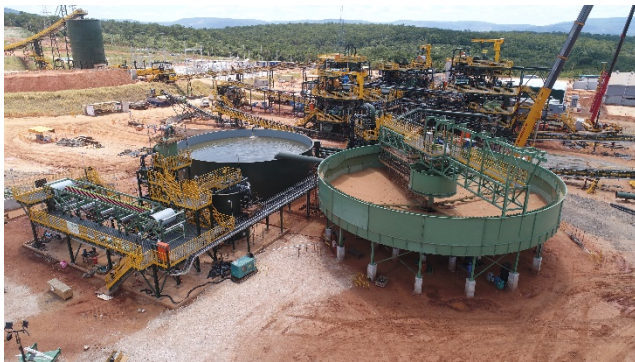
Figure 7: DMS Circuit Commissioning
