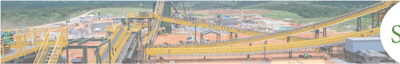
Figure 5: Crushed Ore Bin Area
