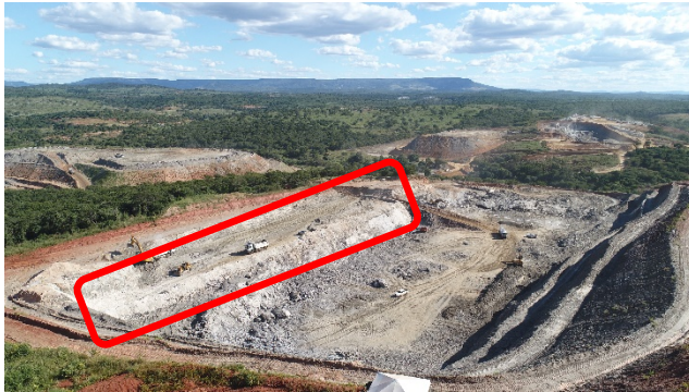
Figure 9: Phase 1 North Pit Mining
