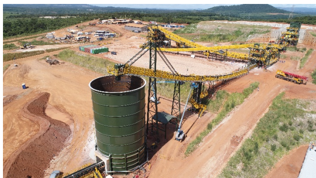
Figure 7: DMS Circuit Commissioning
