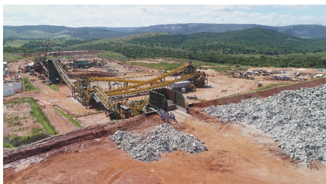
Figure 5: Crushed Ore Bin Area
