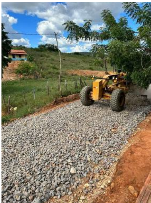
Figures 3 and 4: Coarse gravel tailings being used to pave roads in Vale do Jequitinhonha
