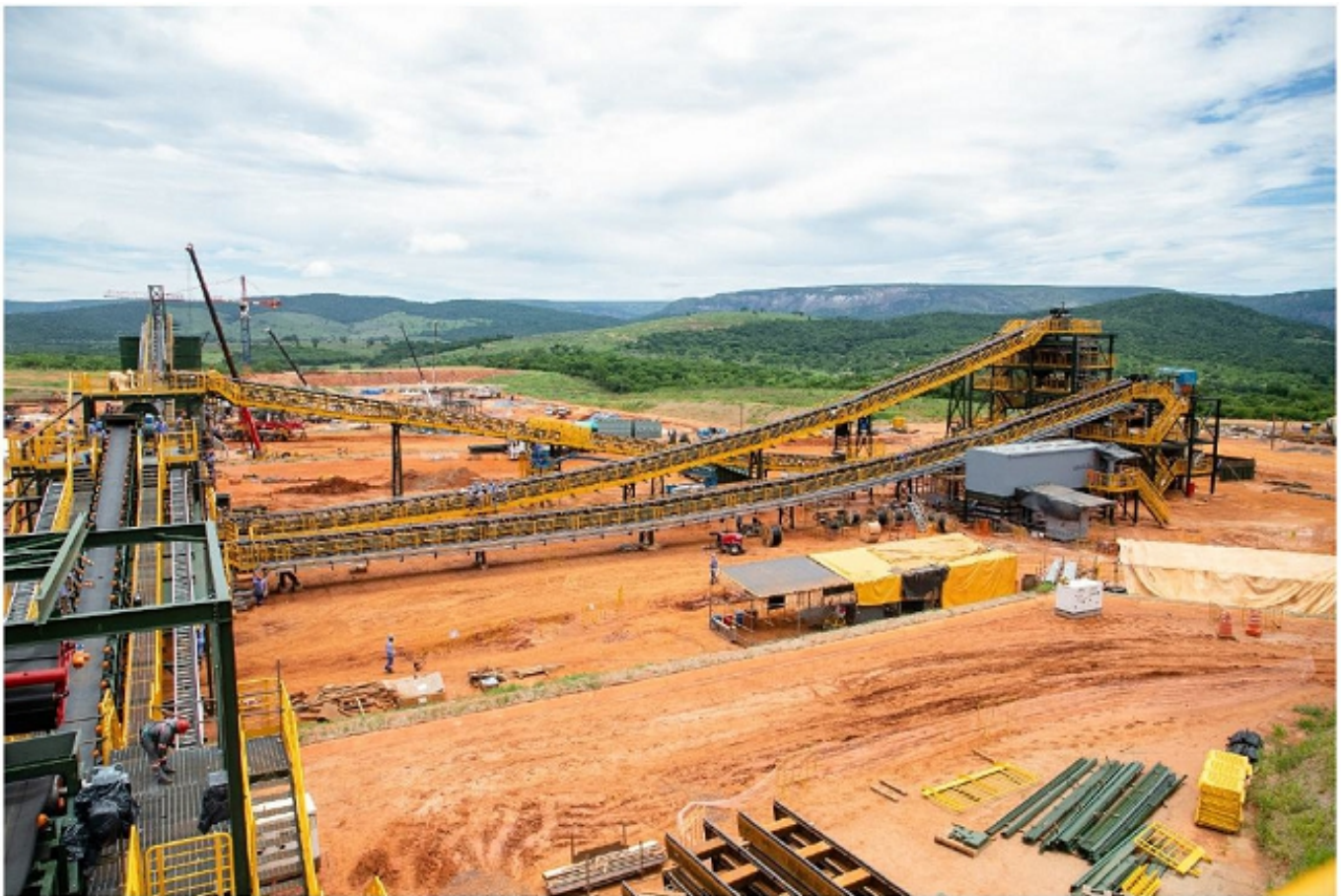
Figure 1: Dry Plant Commissioning Commencement
