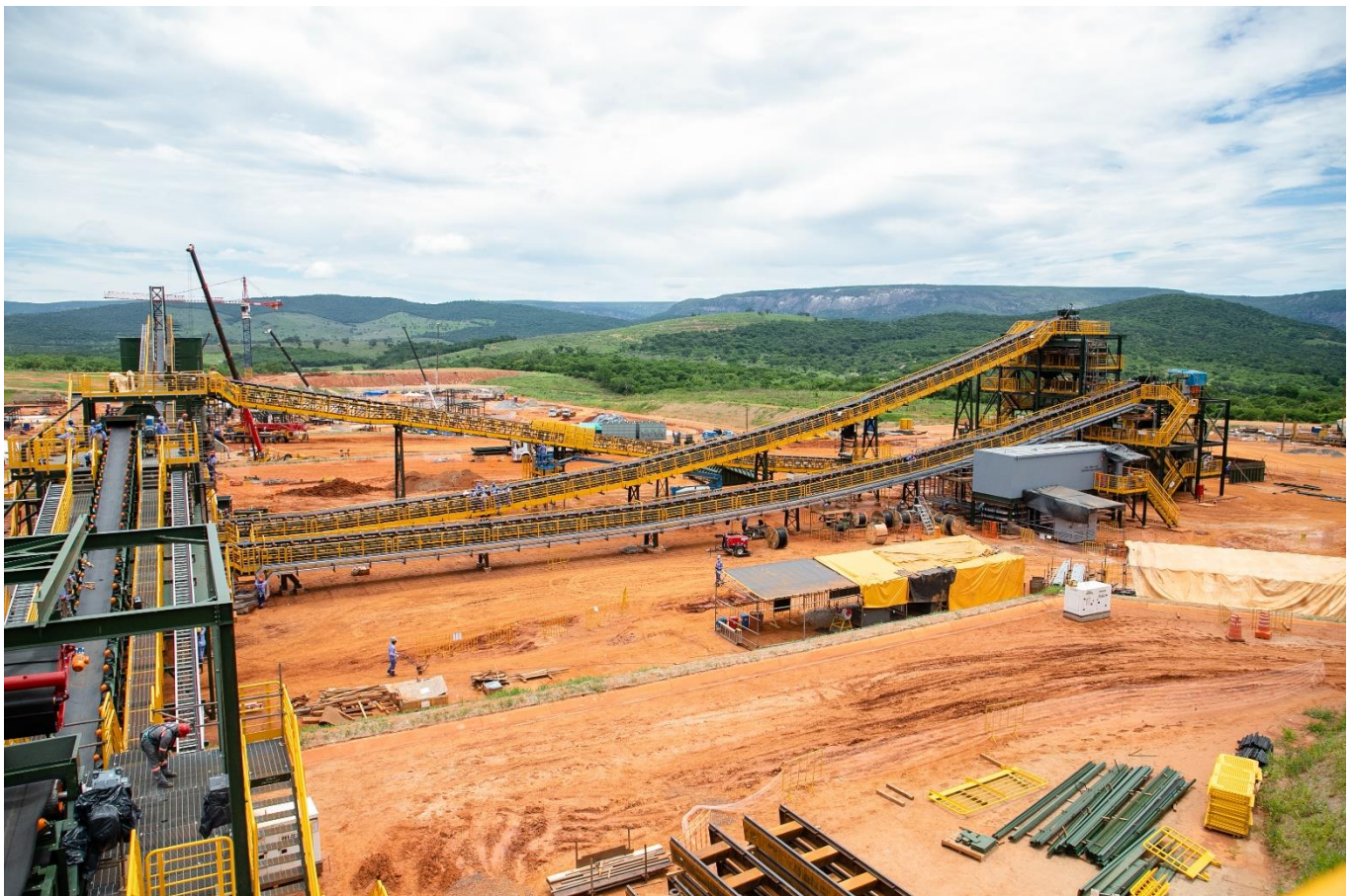
Figure 1: Dry Plant Commissioning Commencement
