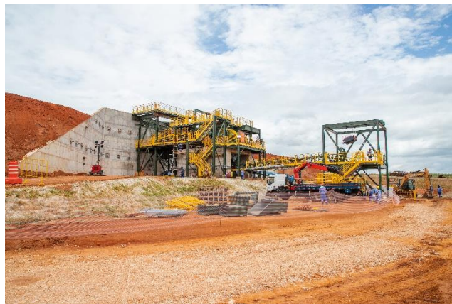
Figure 6: Construction of Crushed Ore Bin Area
