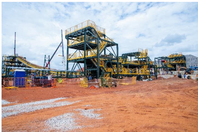
Figure 5: Secondary / Tertiary Crusher Installation
