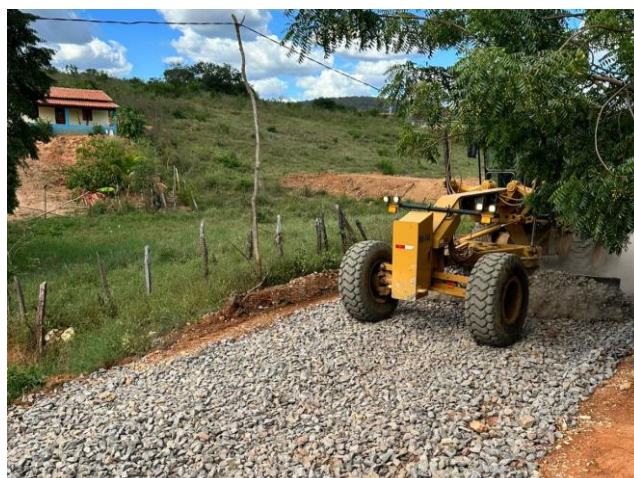
Figure 22: Coarse Gravel Tailings Paving Roads
